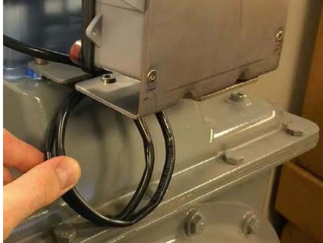
Figure 5 - 17. Coil the Excess Cable
