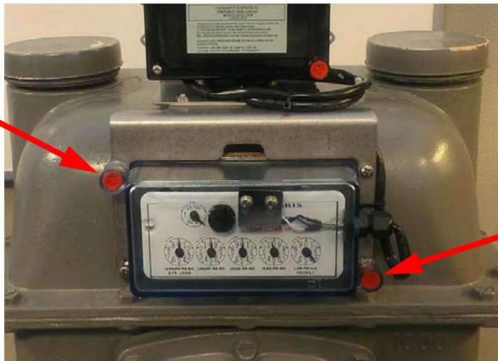
Figure 6 - 25. GPR Assembly installed on a Sprague Large Diaphragm Meter
