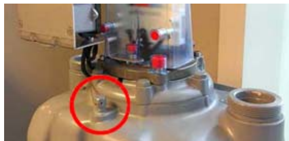
Figure 3 - 25. Meter Pressure Tap
