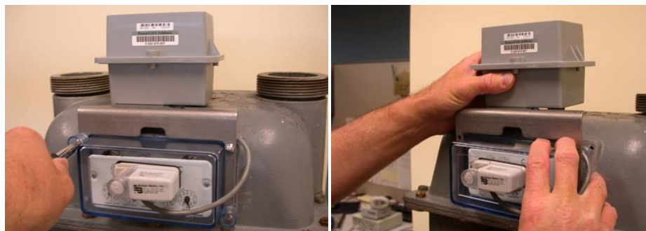
Figure 6 - 2. Remove Tamper Seals and Screws – Carefully Remove Module & Bracket Assembly
