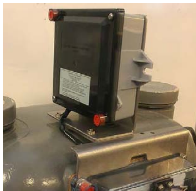
Figure 6 - 27. GPR Facing Left Side of Meter
