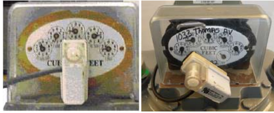
Figure 4 - 3. Center Dial and Offset Dial Mount Rockwell Commercial Index Covers
