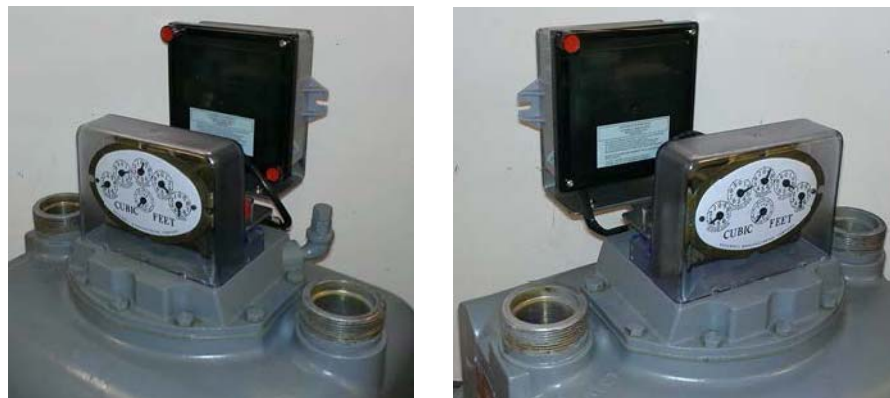
Figure 4 - 19. GPR and Index Cover Installed in Both Orientations
