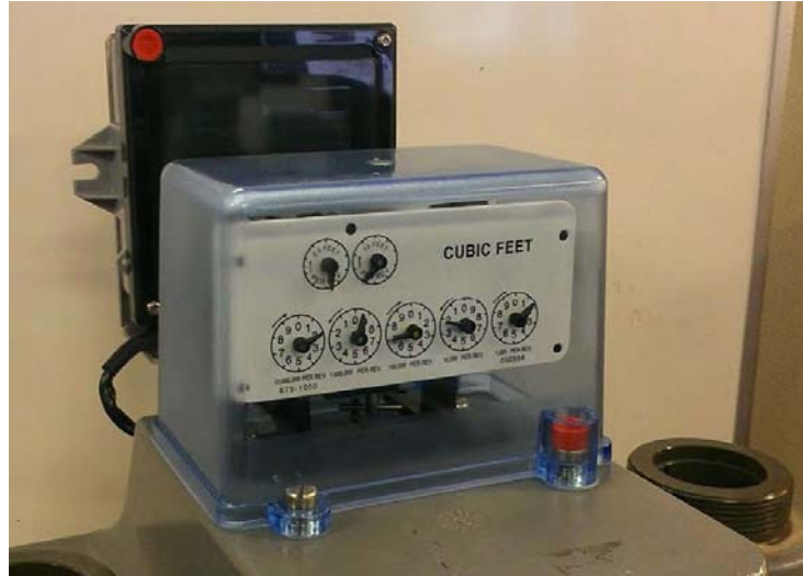
Figure 5 - 19. GPR and Index Cover Assembly Installed On a Schlumberger Large Diaphragm Meter
