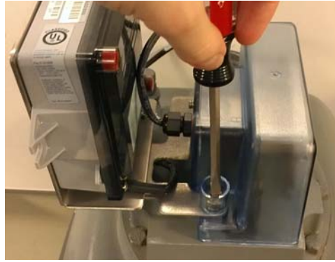
Figure 4 - 15. Tighten Bracket Screws 15 to 20 inch-pounds
