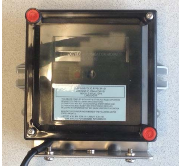
Figure 2 - 8. GPR Installation Complete
