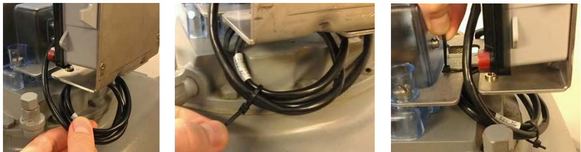
Figure 4 - 16. Coil Excess Cable
