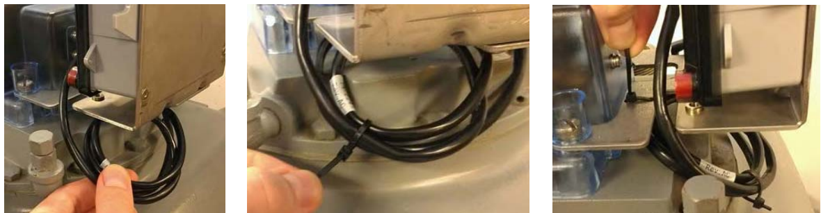
Figure 3 - 16. Coil Excess Cable
