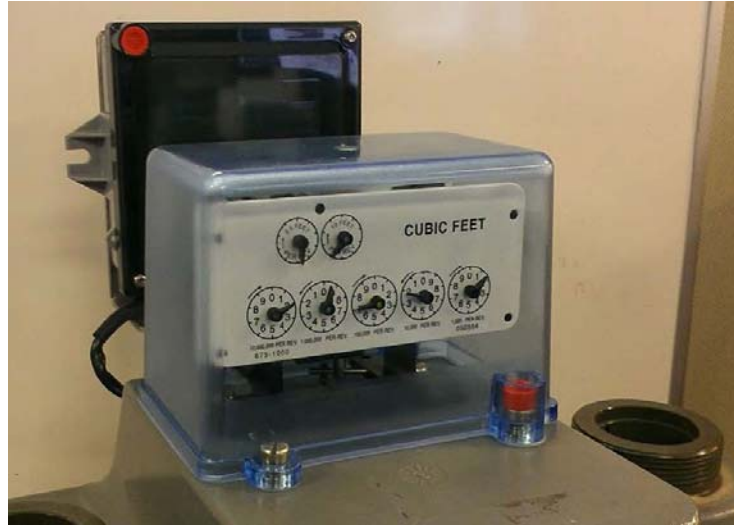
Figure 4 - 19. GPR and Index Cover Assembly Installed On a Schlumberger Large Diaphragm Meter
