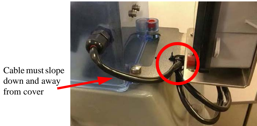
Figure 4 - 18. Route and Attach the Excess Cable
