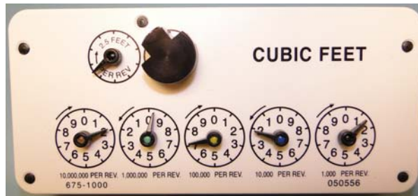
Figure 5 - 16. Balanced Dial Wheel Installed
