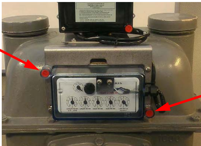
Figure 5 - 25. GPR Assembly installed on a Sprague Large Diaphragm Meter
