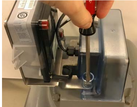
Figure 3 - 15. Tighten Bracket Screws 15 to 20 inch-pounds
