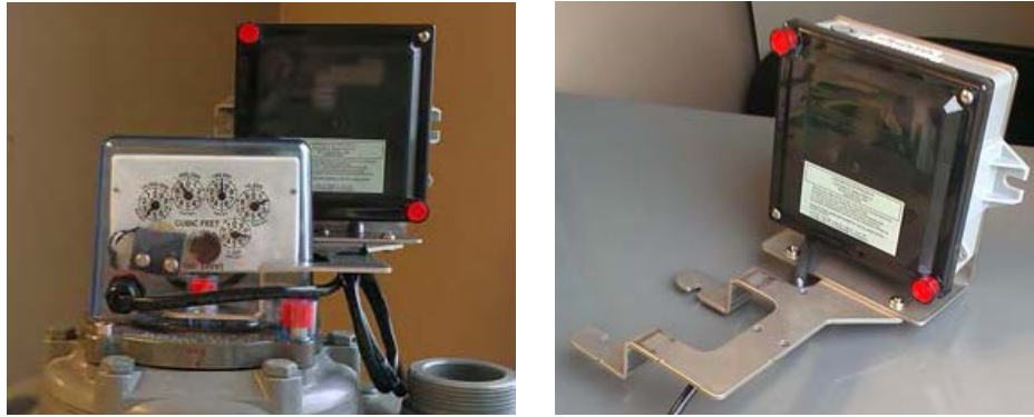
Figure 2 - 31. GPR at Right Rear - Using 28-1440 Bracket
