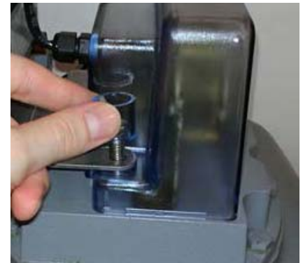
Figure 3 - 14. Install GPR Bracket, Screws and Tamper Cups
