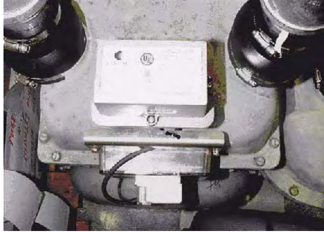
Figure 6.25 Sprague/Actaris: meter with module installed
