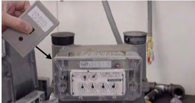
Figure C.3 Sprague/Schlumberger/Actaris RF placement
