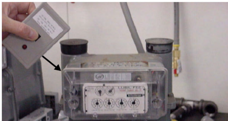
Figure C.3 Sprague/Schlumberger/Actaris RF placement
