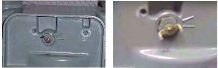
Figure 5.45 Lancaster/National: Installation of New Coupler
