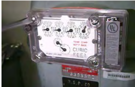
Figure 5.22 Rockwell/Equimeter/Sensus: Installing the Meter Module cover
