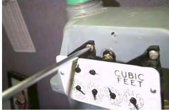
Figure 5.28 Sprague/Schlumberger/Actaris: Removing the index
