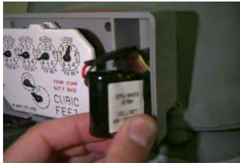
Figure 5.20 Rockwell/Equimeter/Sensus: Correct battery orientation (connector on top)
