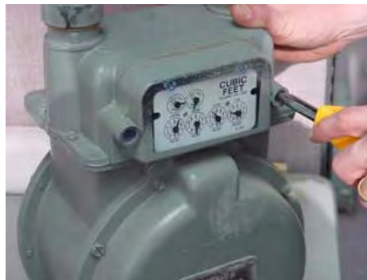
Figure 5.42 Lancaster/National: Removing the index cover
