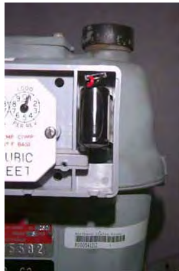
Figure 5.20 Rockwell/Equimeter/Sensus: Correct battery orientation (connector on top)
