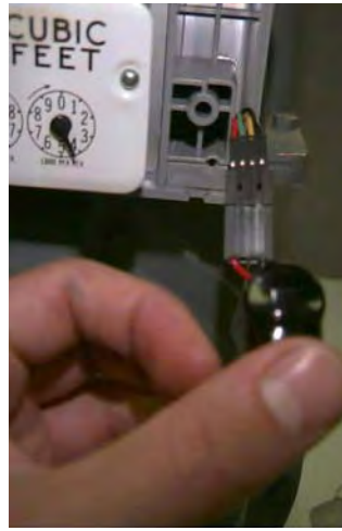
Figure 5.34 Sprague/Schlumberger/Actaris: Connecting the Battery
