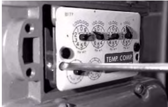
Figure 5.3 American Removing the Index (one screw on each side)
