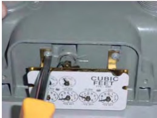
Figure 5.43 Lancaster/National: Removing the index
