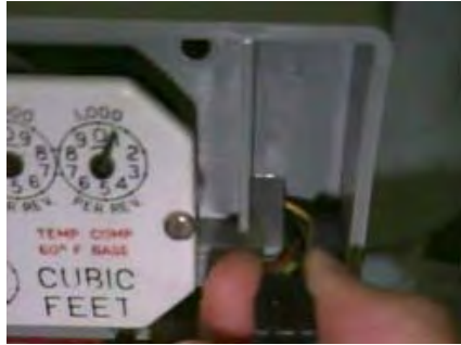
Figure 5.19 Rockwell/Equimeter/Sensus: Connecting the battery
