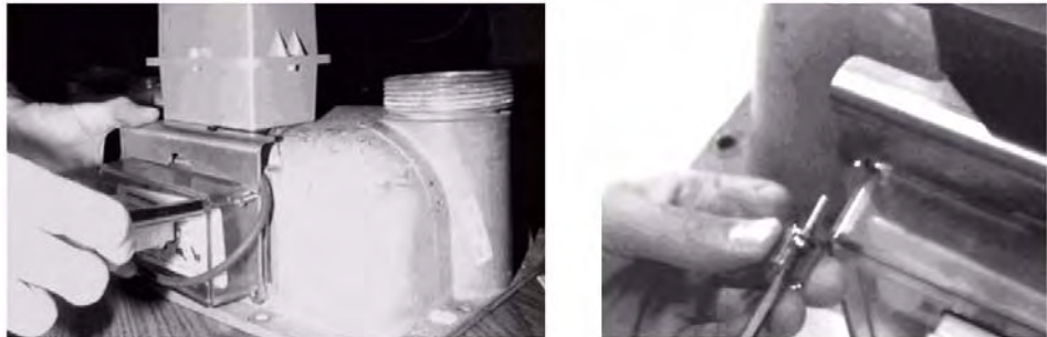
Figure 6.23 Sprague/Actaris: installing Index cover
