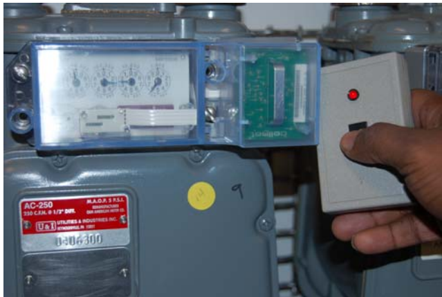
Figure B - 2. Proper Placement of the RF Buster
