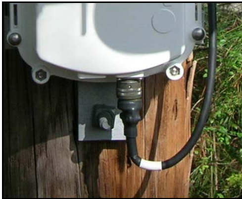
Figure 3 - 1. Cable with a drip loop
