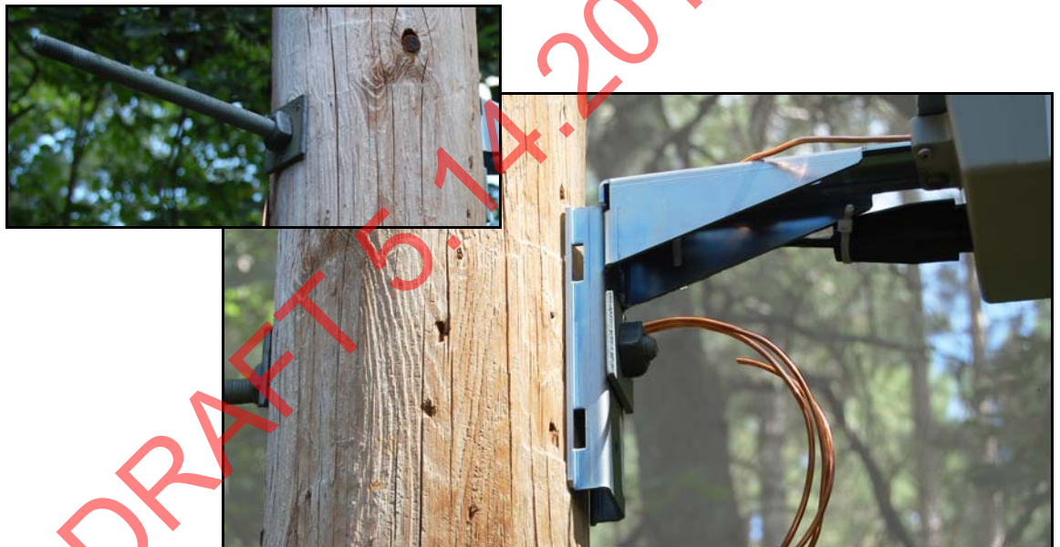
Figure 2 - 5. Attach Mounting Bracket to Wood Pole
