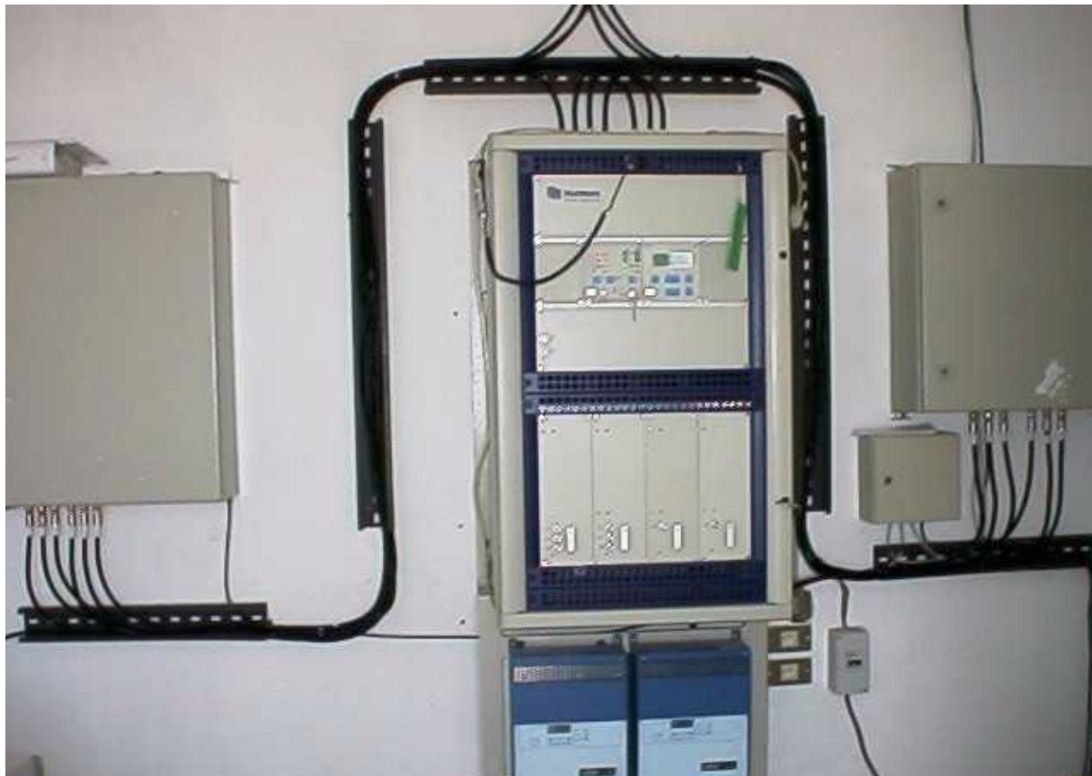
Figure1-4 Localizer Cabinet Installation
