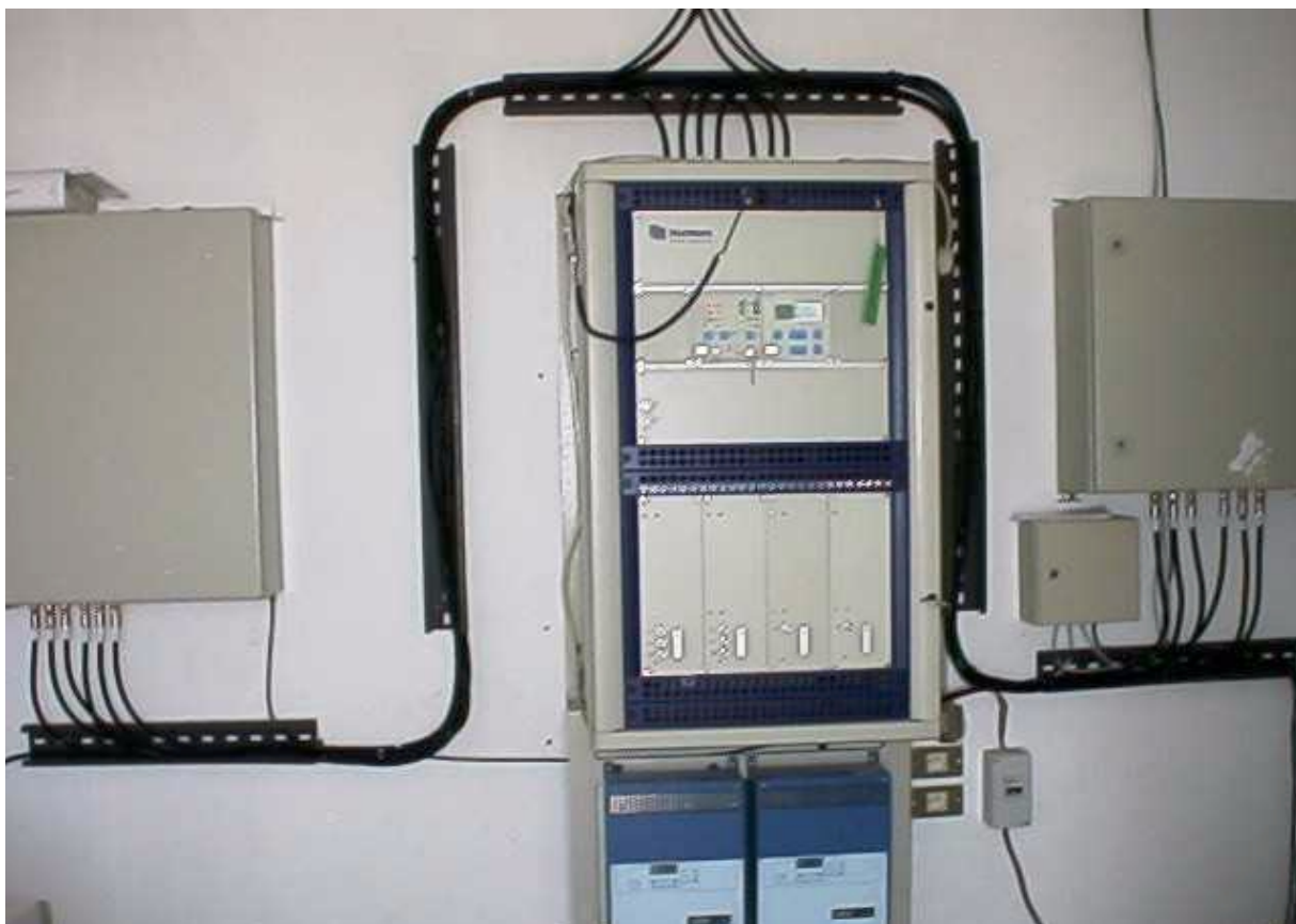
Figure 1-4 Localizer Cabinet Installation
