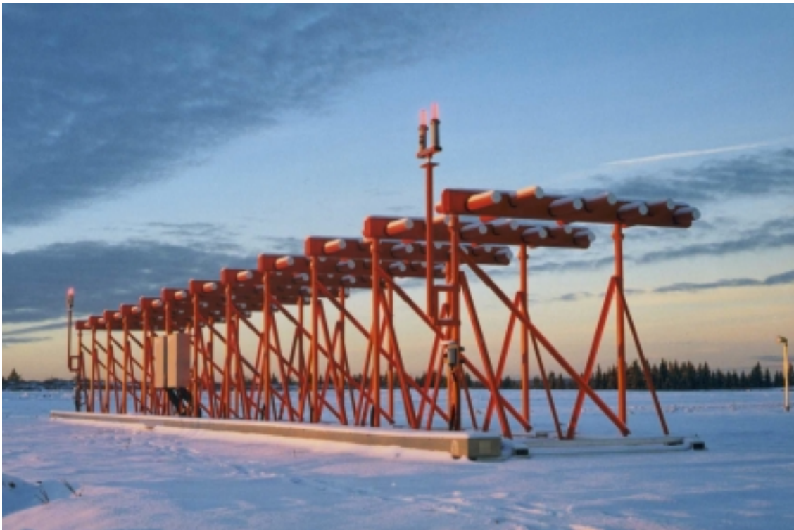
Figure 1-3 Localizer Antenna
