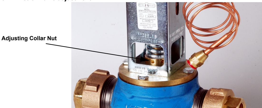
Figure 11 Metrex valve adjustment
