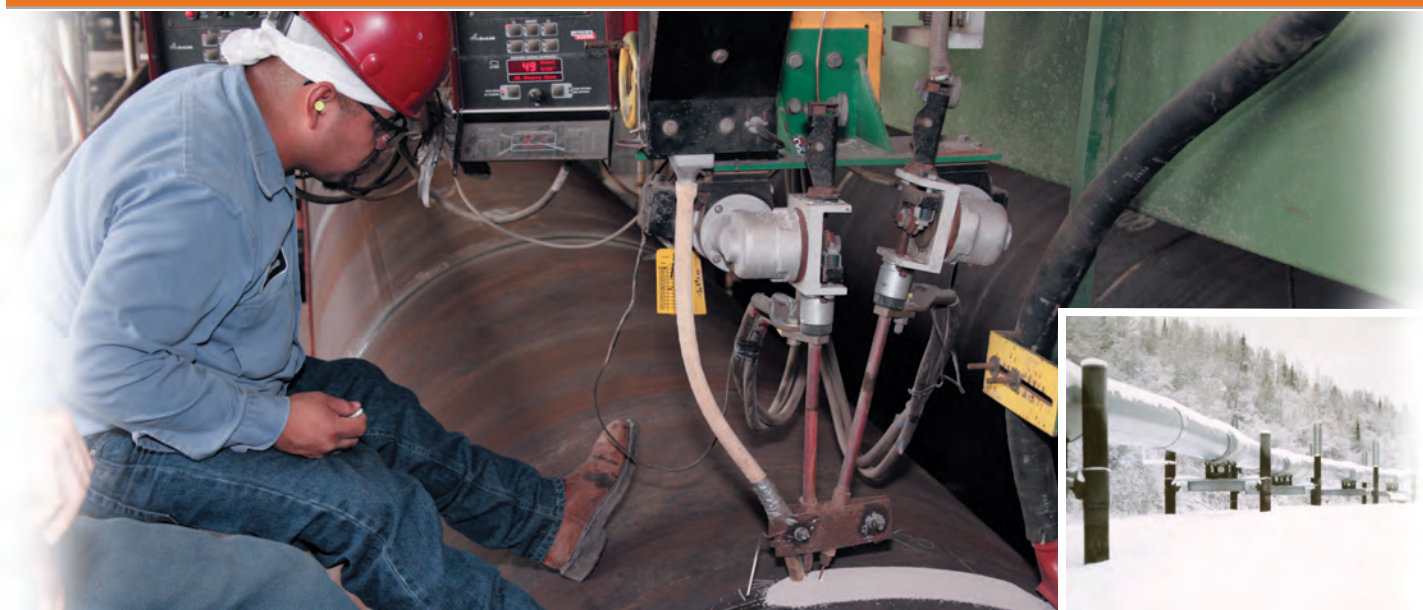
Submerged arc welding with Power Wave® AC/DC 1000 and Power Feed™ 10A Controller.
