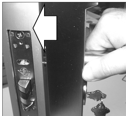
Fig. 8: Install lock onto the door
