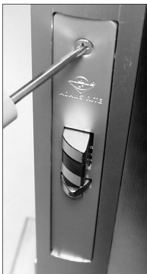
Fig. 7b: Install the latch face plate
