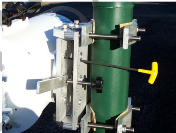
Figure 9. Tighten radio mount screws with 3/16" Allen wrench.
