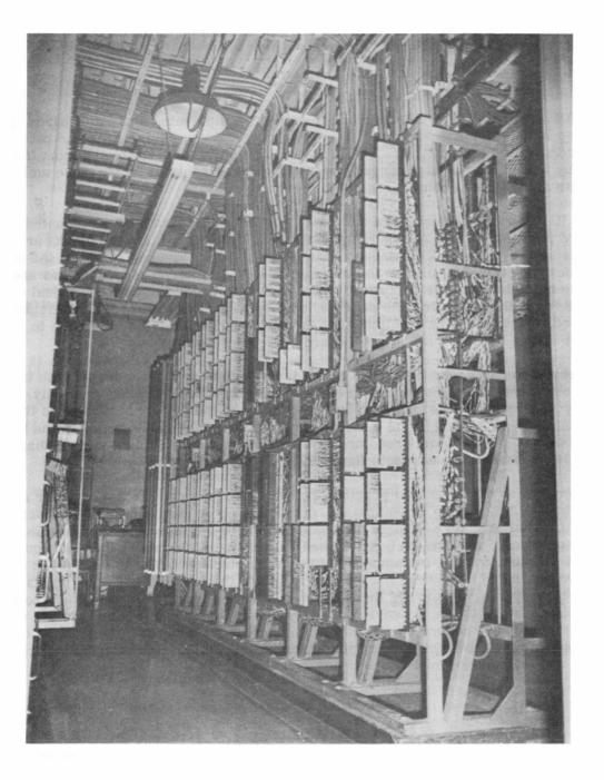
Figure 9-5. Typical Main Distribution Frame
