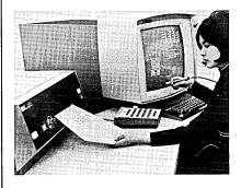
The 2285, shown at the left, can produce a photo copy in 15 to 38 seconds, depending on the complexity of the image. When the "copy" button on the 2285 is pushed, the signals that produce the display on the large screen are transferred to a small cathode-ray tube (CRT) in the copier. The CRT's image is projected onto  $8\frac{1}{2}$ " by 11" photo-sensitive paper.
