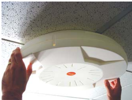
Figure 44. Attaching the Unit (XS-3900)
