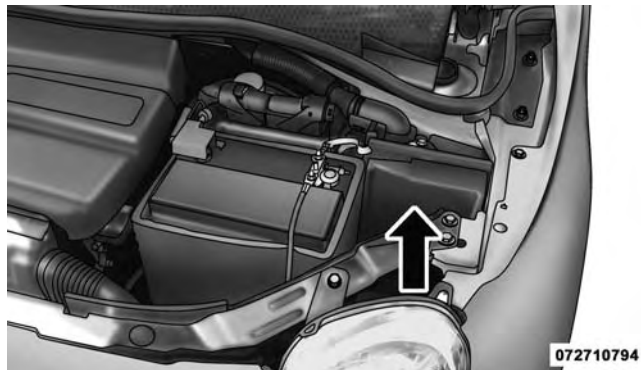
Front Distribution Unit
