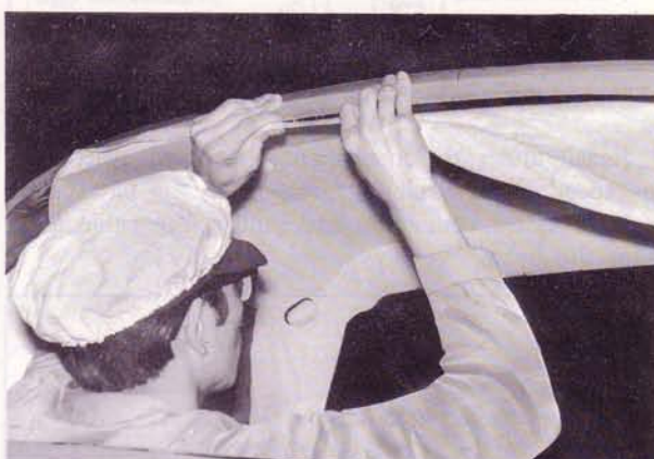
Fig. 14-16 Gluing headlining
