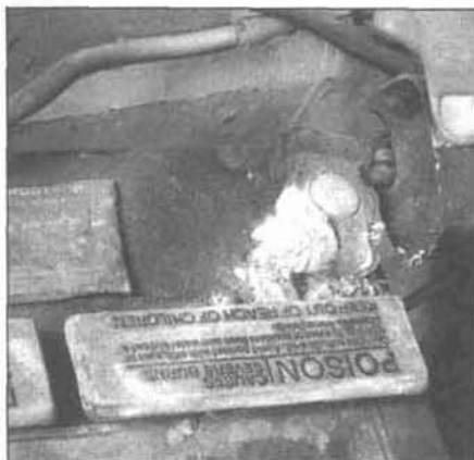
6.6a Battery terminal corrosion usually appears as light, fluffy powder
