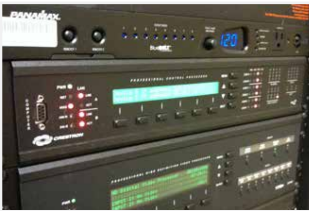
Panamax BlueBOLT-enabled M4315-PRO’s are integrated with Crestron Control Systems at SLU to facilitate local and remote power control and monitoring.
