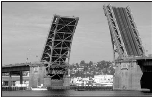
Fig. 52 Bascule Bridge opening for shipping.
