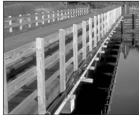
Fig. 2 - Simple beam bridge.
