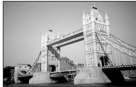
Tower Bridge, London, England.
