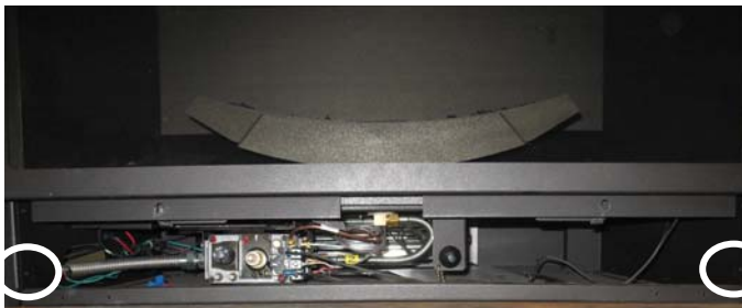
Faceplate secured to inner side of firebox flange.
