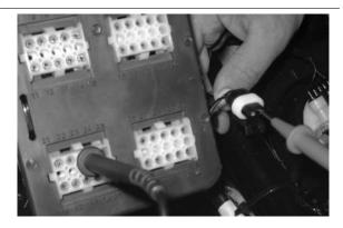
12 - Check the earth insulation of the negative line.
