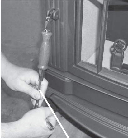
Secure using 7/16" socket wrench.
