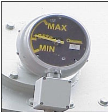
Figure 28 – Conservator Oil Level.
