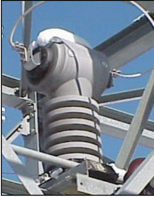
Current Transformer in Switchyard.
