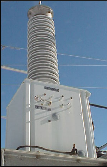
Potential Transformer in switchyard.
