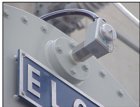
Figure 41 – Photograph of a Bladder Failure Relay.
