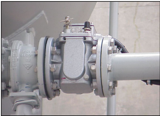
Figure 34 – Photograph of a Buchholz Relay.
