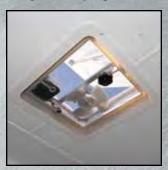
Roof Vent with Exhaust Fan
