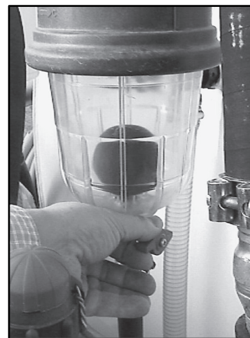
Figure 3.3 Moisture Trap Drain Valve
