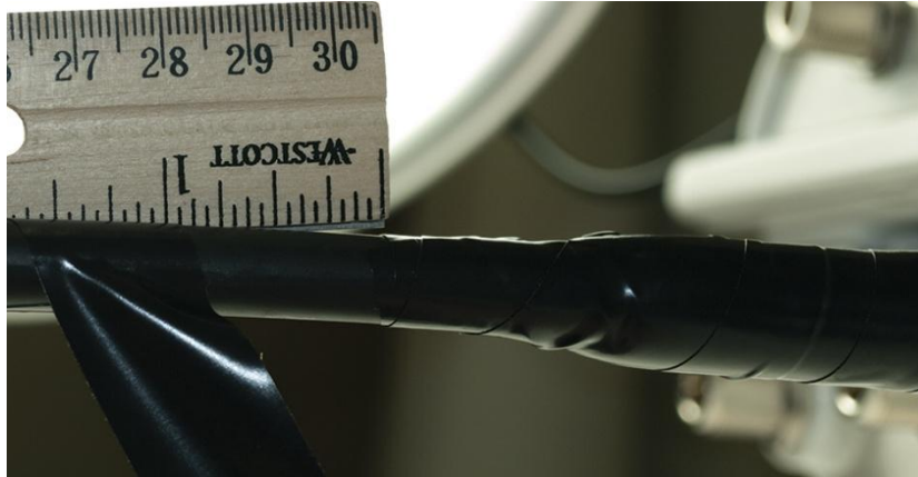
Figure 37: Wrapping \frac{3}{4} " Plastic Tape 1" Below Previous Wrap
