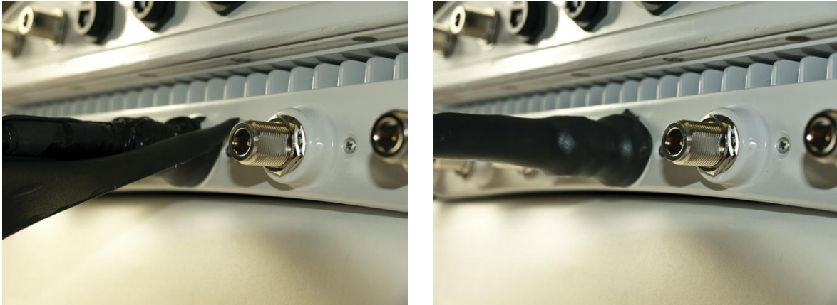
Figure 35: First Rubber Tape Layer
