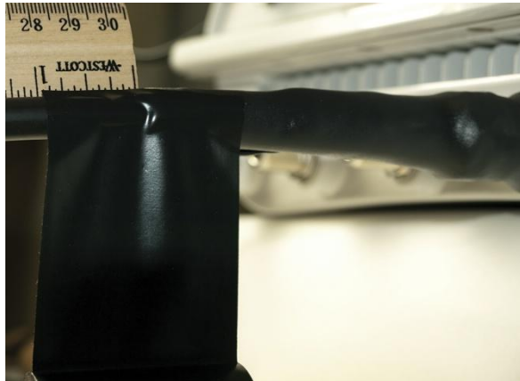
Figure 36: Wrapping Plastic Tape on Top of the Rubber Tape
