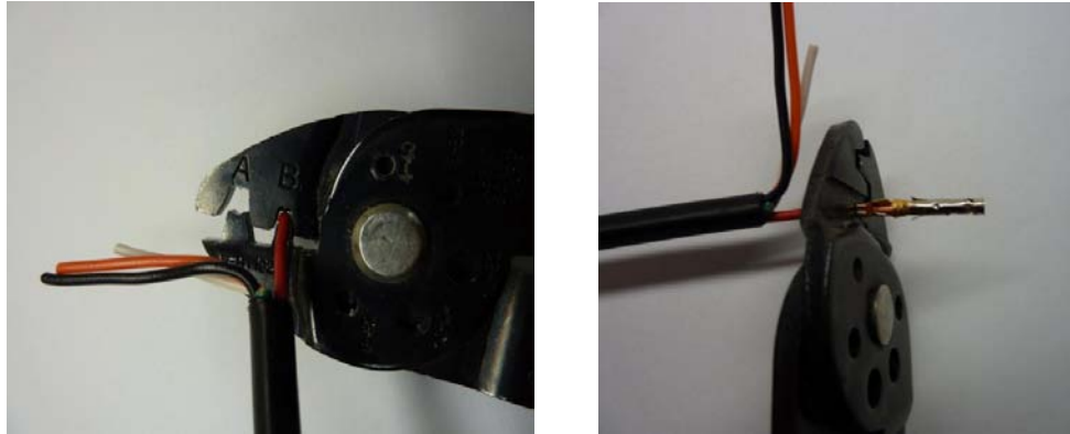
Figure 22: Side and top views of correct crimping technique
