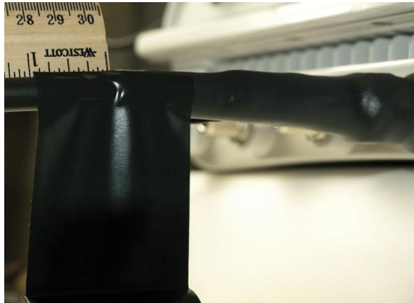
Figure 37: Wrapping Plastic Tape on Top of the Rubber Tape
