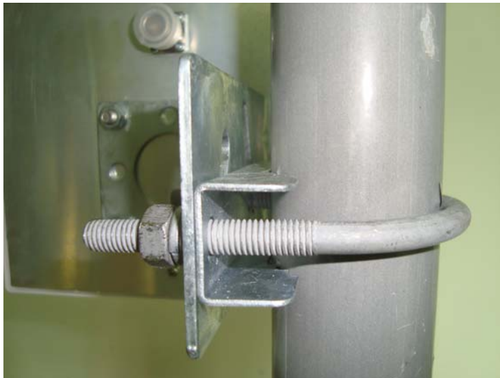
Figure 59: L-Bracket Attached to Pole
