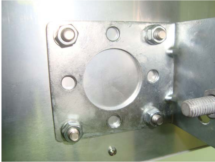
Figure 59: L-Bracket Attached to Pole
