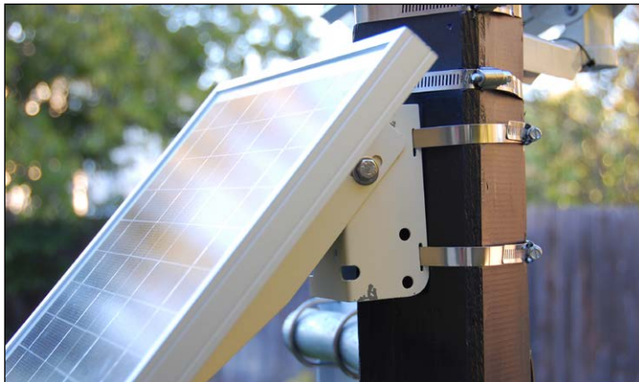
Solar panel mounted to a pole using stainless steel hose clamps that are passed through the slots in the bracket. This allows for a quick, non-permanent installation that may be easily relocated, without damaging the mounting surface.
