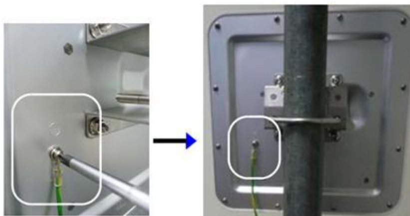
Figure 6-2 Attach the Ground Cable to the ODU
