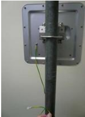
Figure 6-3 AttachGround Cable to the Ground
