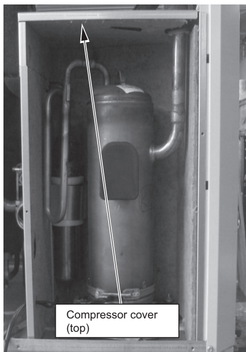
4. Remove the compressor cover (top).
