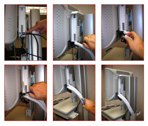
13. Pull the excess cable length to the bottom of the column
