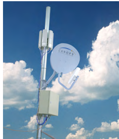
Figure 13: CMM2 pole-mounted
