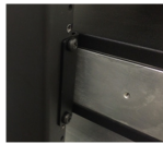
Figure 1b: Rack installation
