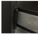
Figure 1b: Rack installation
