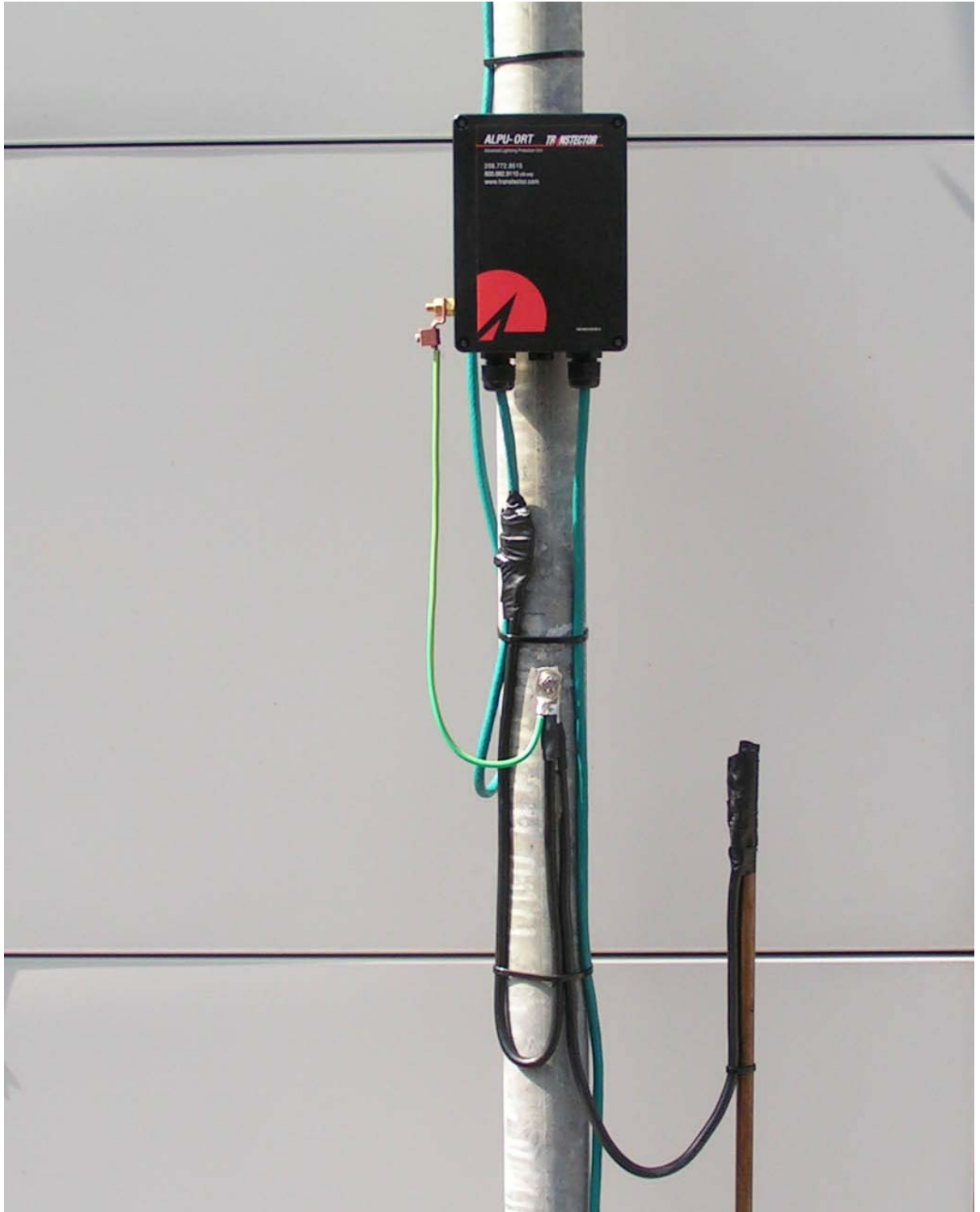
Figure 97 - Lower Grounding Configuration
