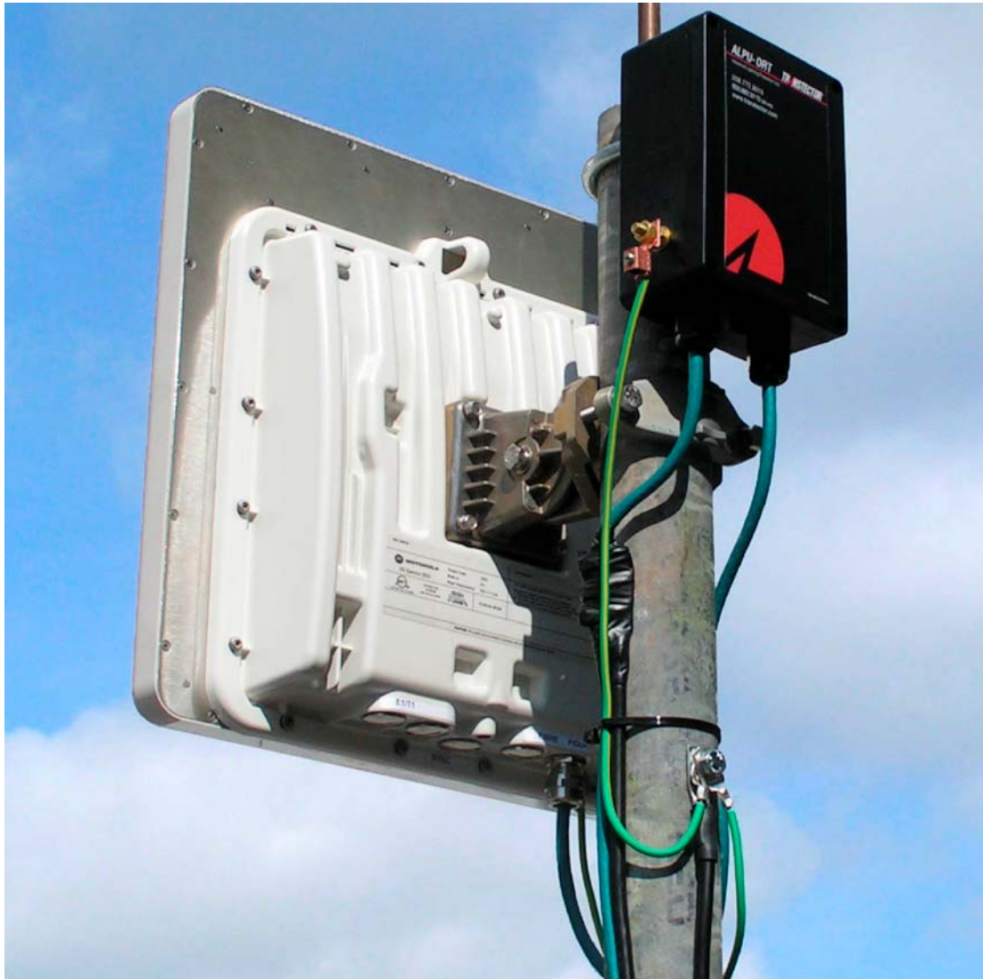
Figure 79 - Upper Grounding Configuration
