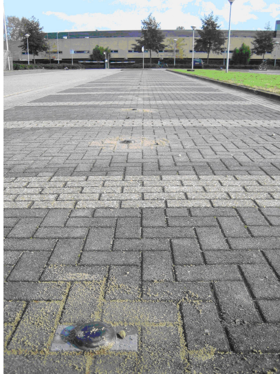
Figure 6: Finished SENSIT installation
