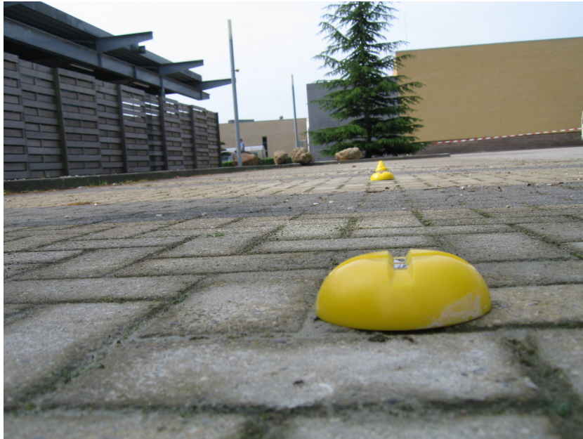
Figure 6: Finished SENSIT IR installation
