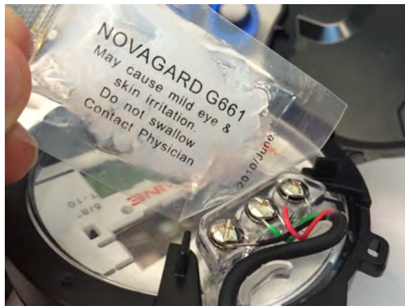
Figure 8 – Application of the Sealant
