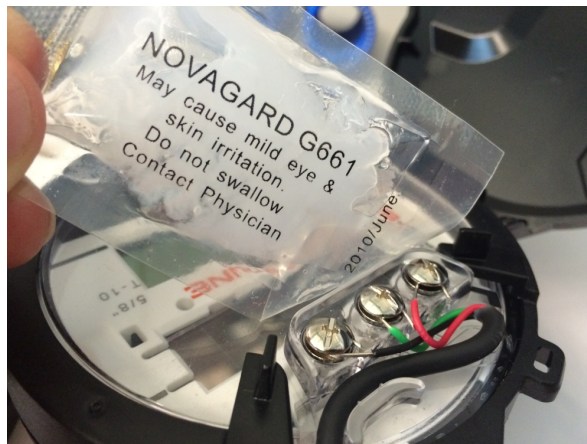
Figure 11 – Application of the Sealant
