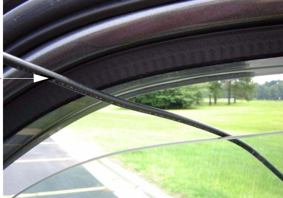
Figure 3.9 Antenna Cable Through Window
