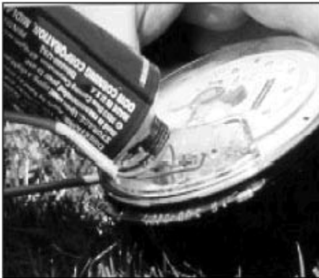
Figure 2.6 Installing Moisture Protection Compound
