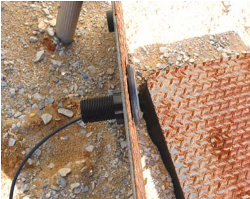
Figure 12 Inserting Antenna into the Pit Lid
