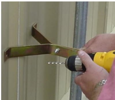
Figure 45 – Lining Up Second Bracket
