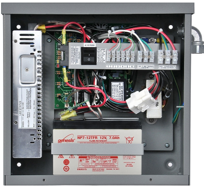
Figure 34 – Wire Input and Output Connectors
