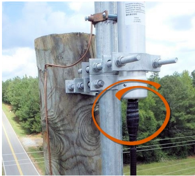
Figure 47 – Weatherizing the RF Antenna Connection
