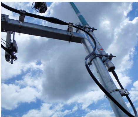
Figure 46 – RF 450 MHz Antenna Connection
