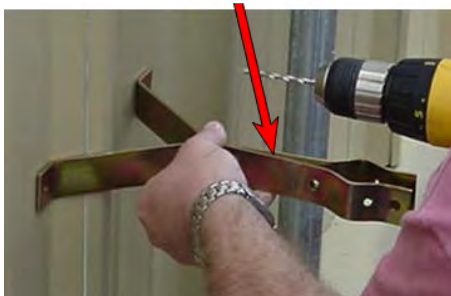
Figure 54 – Securing the Pole Bracket
