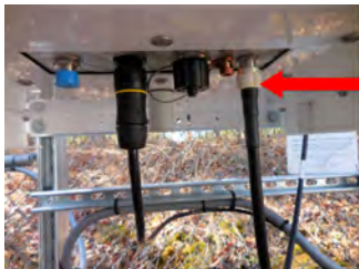
Figure 14 – Cellular Antenna Connection at Base
