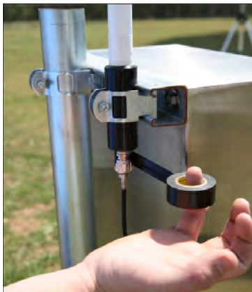
Figure 15 – Weatherizing Connections
