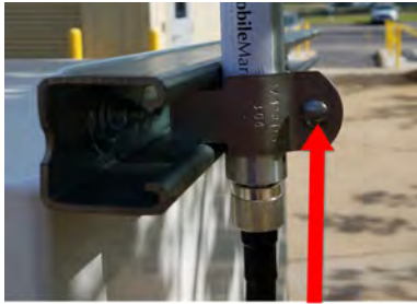
Strut clamp bolt
