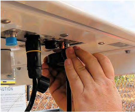
Figure 16 – Weatherizing the Base Connection
