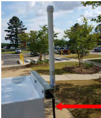
Figure 13 – Cable to Cellular Antenna
