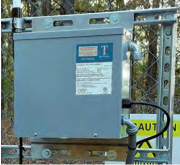
Figure 37 – Strut Channel or Wall Mounting
