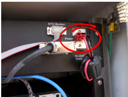
Figure 45 – Radio Modem Power Front Panel Connector
