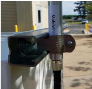
Figure 11 – Attaching the Cellular Antenna
